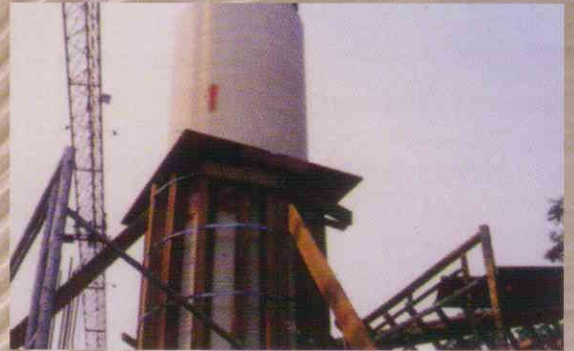
COLUMN FORMWORK
